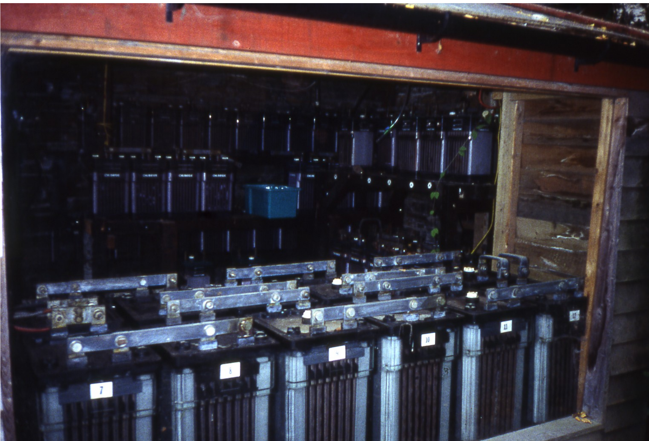
Part of battery bank, Centre for Alternative Technology, Wales
