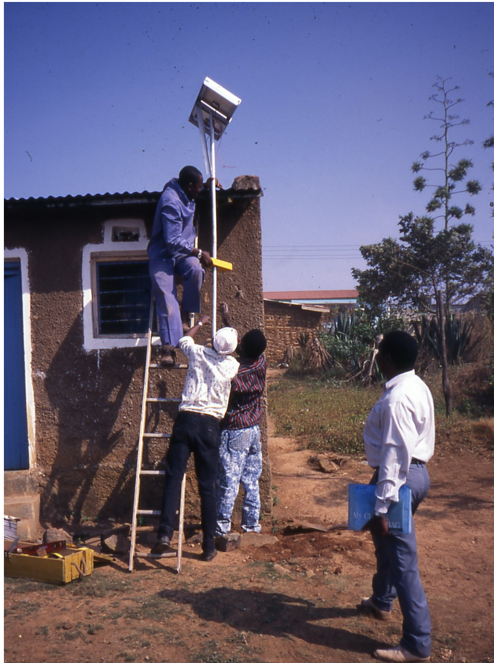
Installing a small solar home lighting system, Tanzania
