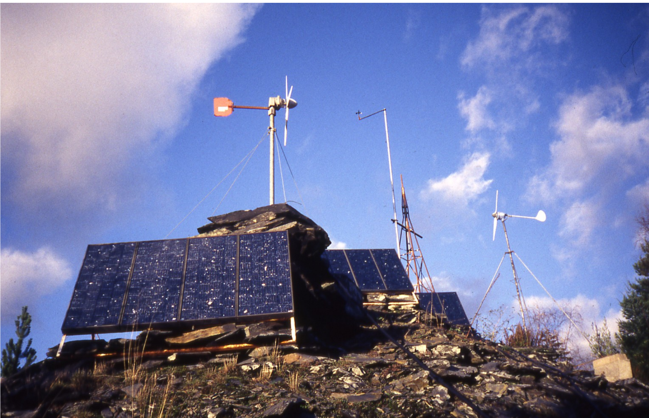
Solar-wind hybrid system, Centre for Alternative Technology, Wales
