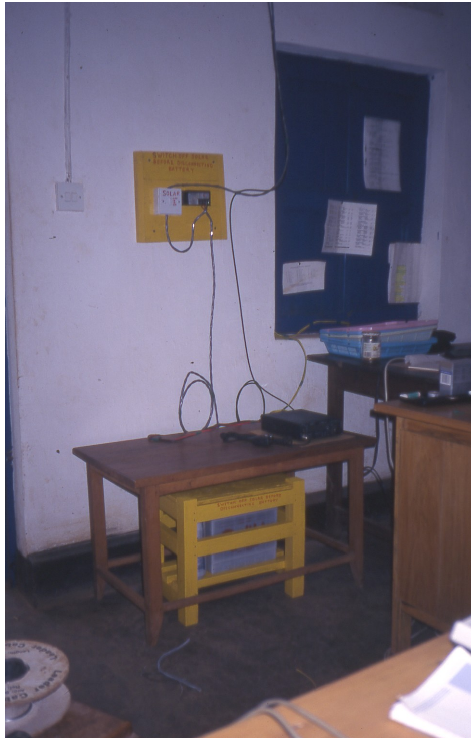
Battery box for two-way radio, Tanzania
