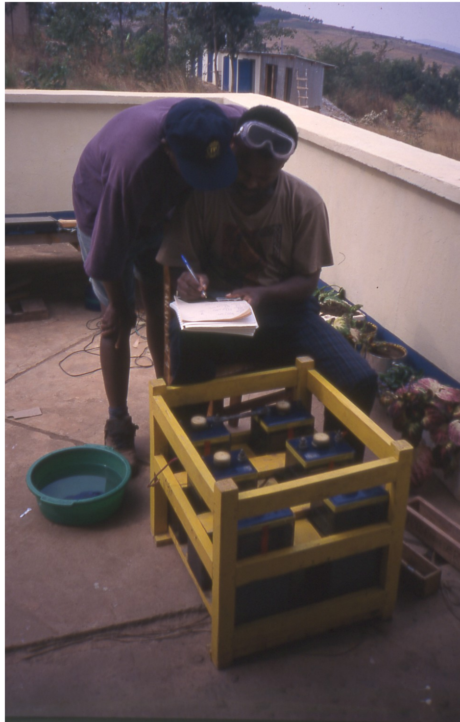
Battery box for school lighting system reconditioned batteries, Tanzania
