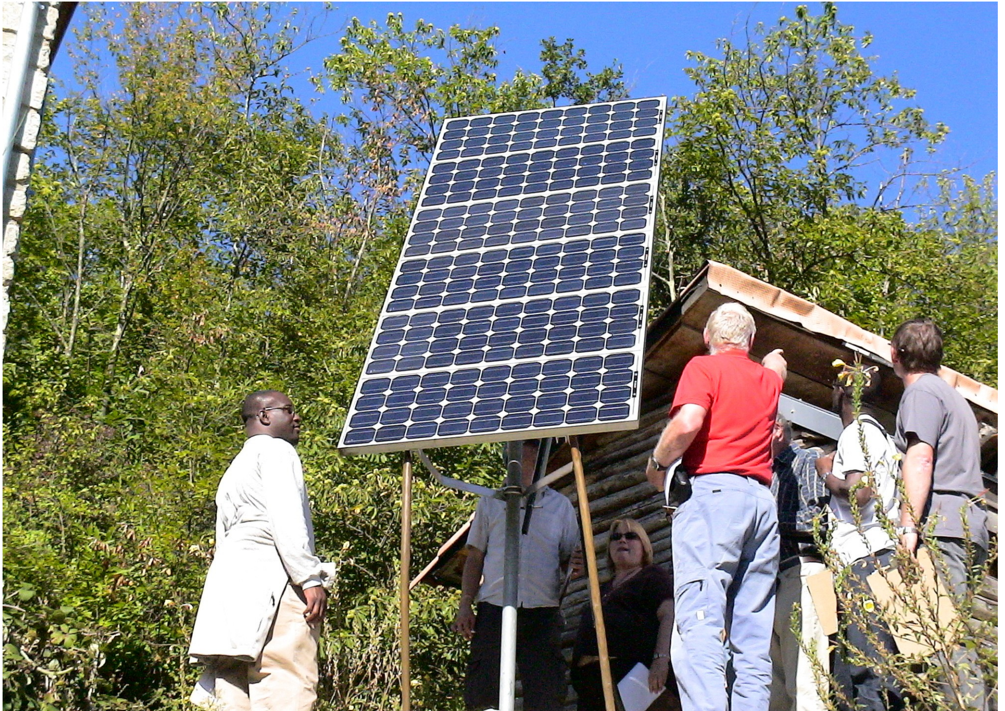
Manual tracking module mount, France
