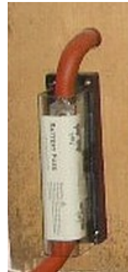
Outback inverter- battery fuse
