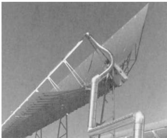
Figure 7.9.1 Collector with linear parabolic concentrator used in a power generation installation. Photo courtesy of Luz Corporation.
