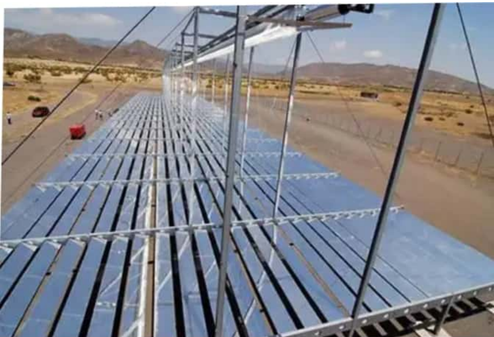
Linear Fresnel Solar Collector
