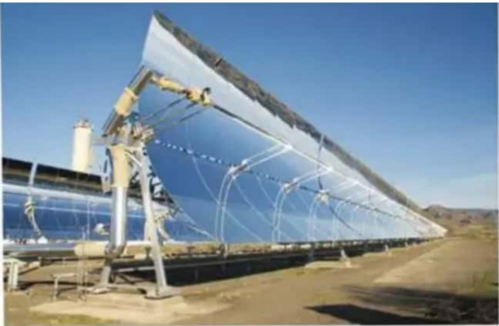
Parabolic Trough Solar Collector
