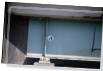
The large shear force that occurs at the support of this steel beam caused localized buckling of the beam's web. To avoid this, a "stiffener" is placed along the web to maintain its shape.
