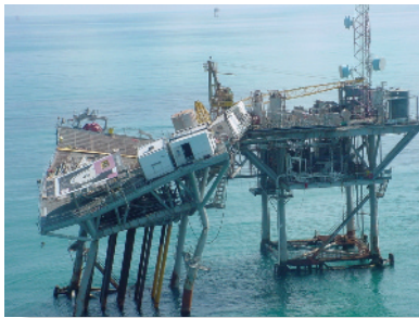
The dramatic failure of this off-shore oil platform was caused by the horizontal forces of hurricane winds, which led to buckling of its supporting columns.
