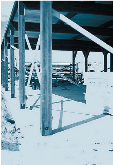
These timber columns can be considered pinned at their bottom and fixed connected to the beams at their top.
