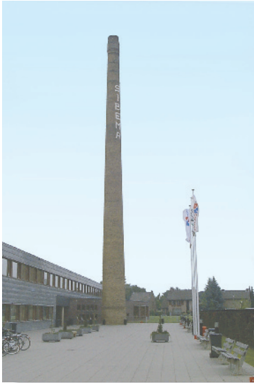
This chimney is subjected to the combined internal loading caused by the wind and the chimney's weight.
