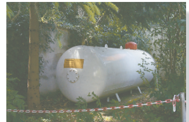
Cylindrical pressure vessels, such as this gas tank, have semispherical end caps rather than flat ones in order to reduce the stress in the tank.
