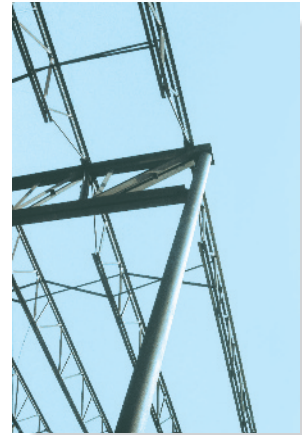
Typical example of a column used to support an eccentric roof loading.
